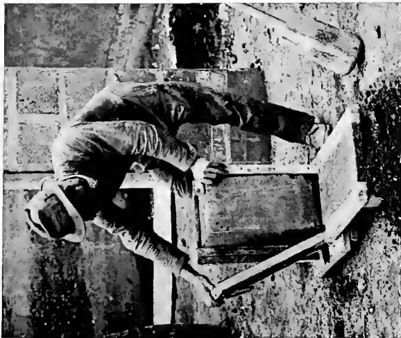
A SIMPLE MOULD FOR PISÉ BLOCKS.
